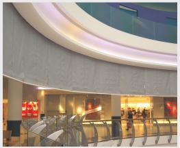
with a white polycarbonate extrusion cover, is used to ensure the curtain deploys under gravity in a controlled manner (Gravity Fail Safe). Heavier bottom bars may be required for some curtains to ensure correct deployment or to reduce deflection of the curtain due to variations in air pressure.
